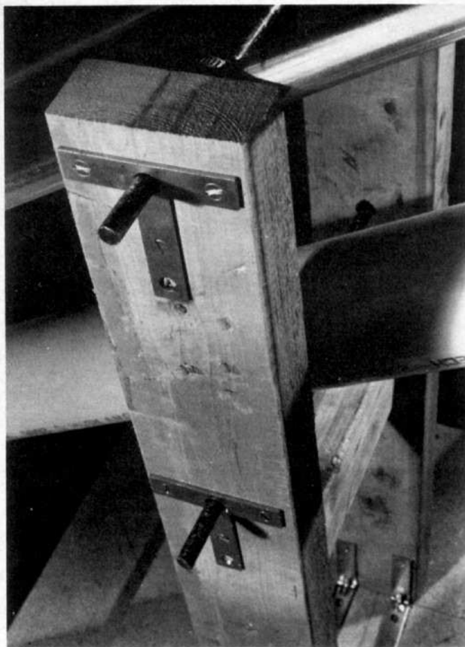
The mending plates and steel rods are aligned vertically on the support posts.
